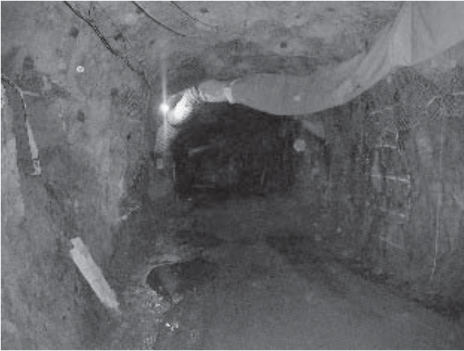
Fig. 3. Digital photograph of the underground gallery.
